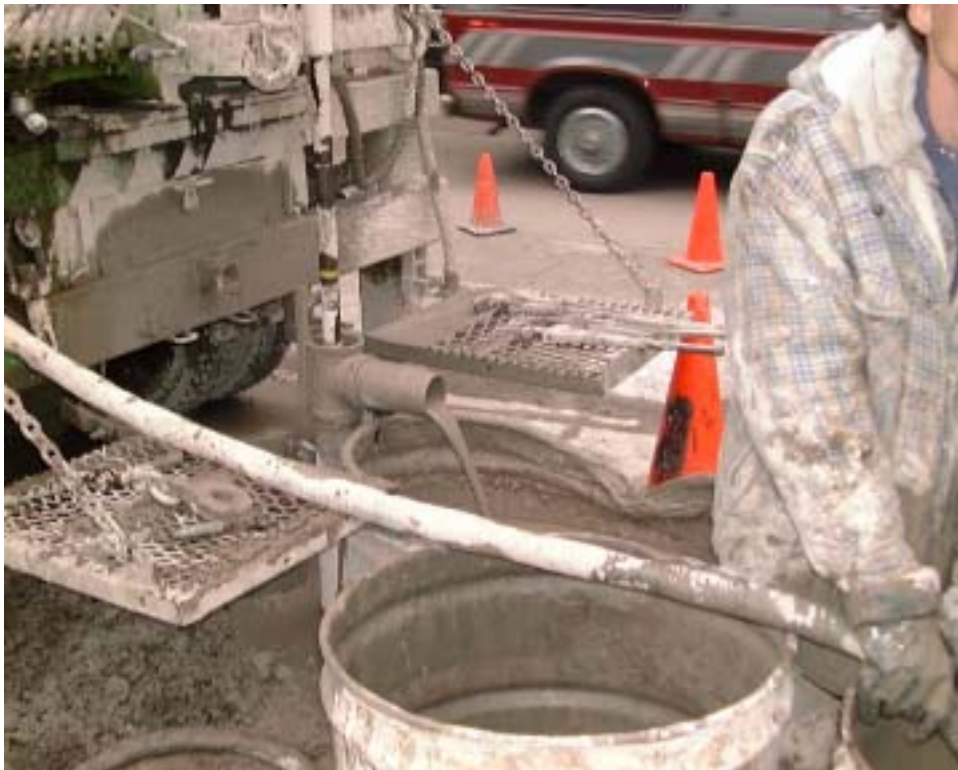
Grout mixing and pumping into a TDR hole
