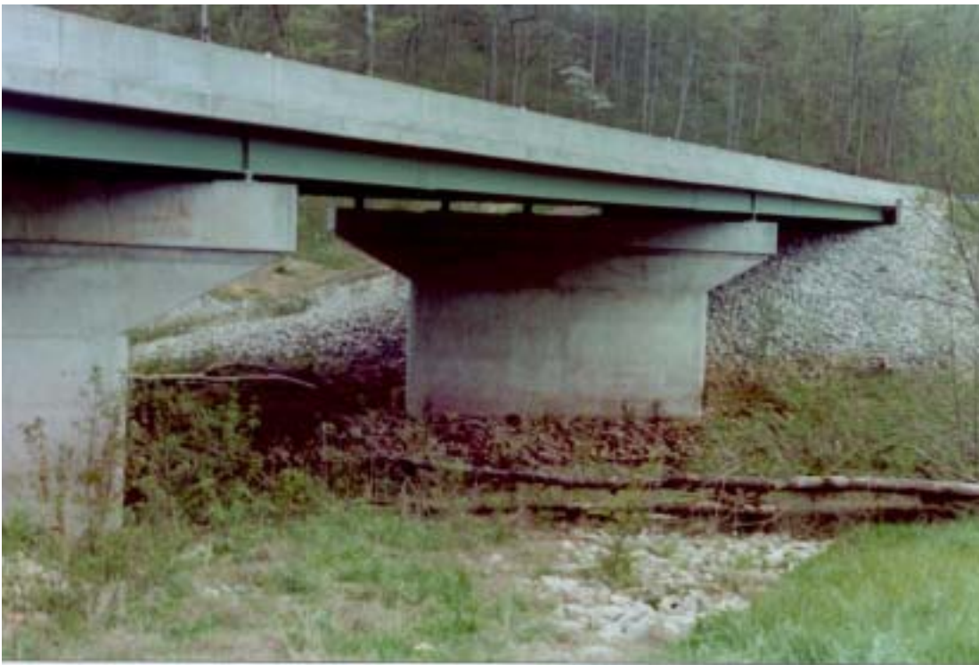
Figure 2-1: View of S.R. 62 bridge over Little Blue River, Crawford County, IN.
