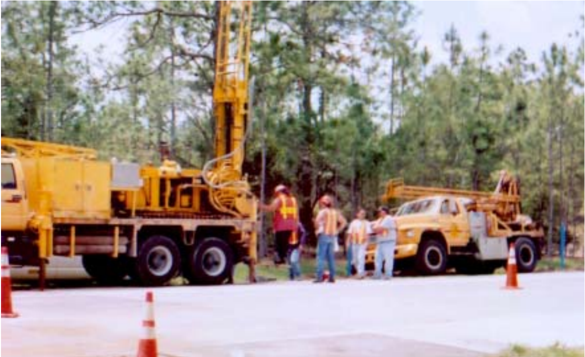
Figure 4-3: Drilling TDR 1 hole at SR.66 site, Florida.
