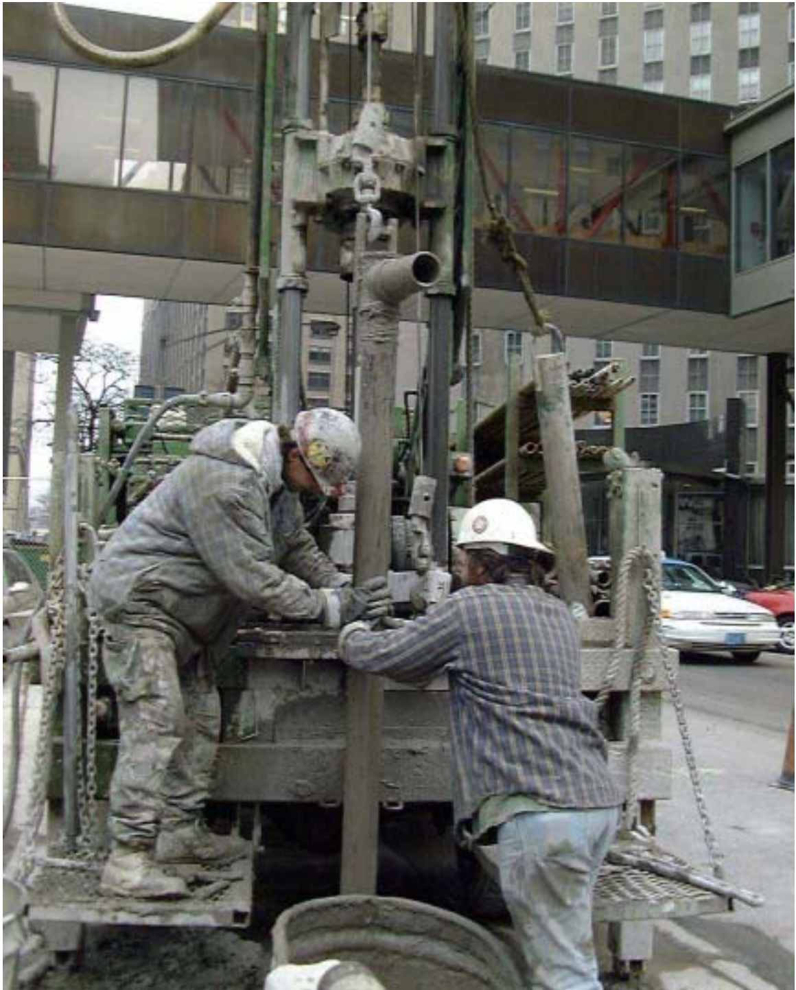
Casing removal for TDR hole drilling
