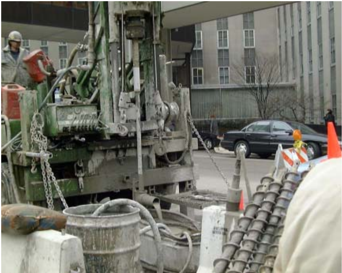
Rotary drilling of TDR hole under bentonite slurry
