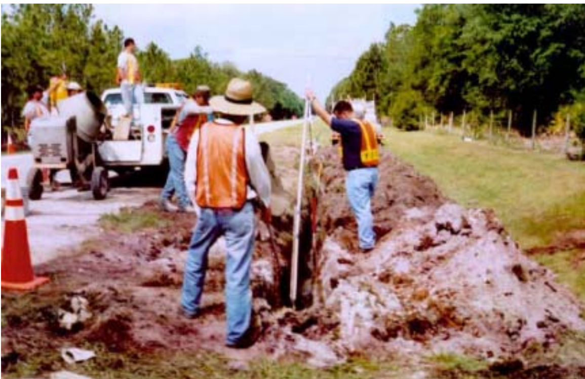
Figure 4-3: Drilling TDR 1 hole at SR.66 site, Florida.
