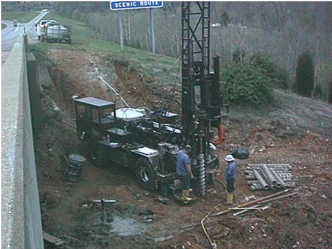
Figure 3-11: View of the pad built for the drilling rig on the west bank of the Little Blue River, Indiana and the drilling of hole B-1-TDR with a hollow stem auger.
