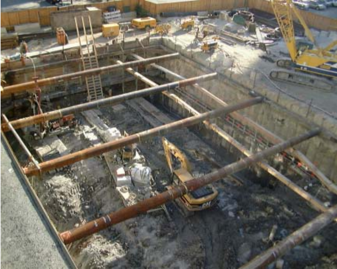
Figure 5-3: Aerial view of the Chicago and State subway excavation, Chicago, Illinois
