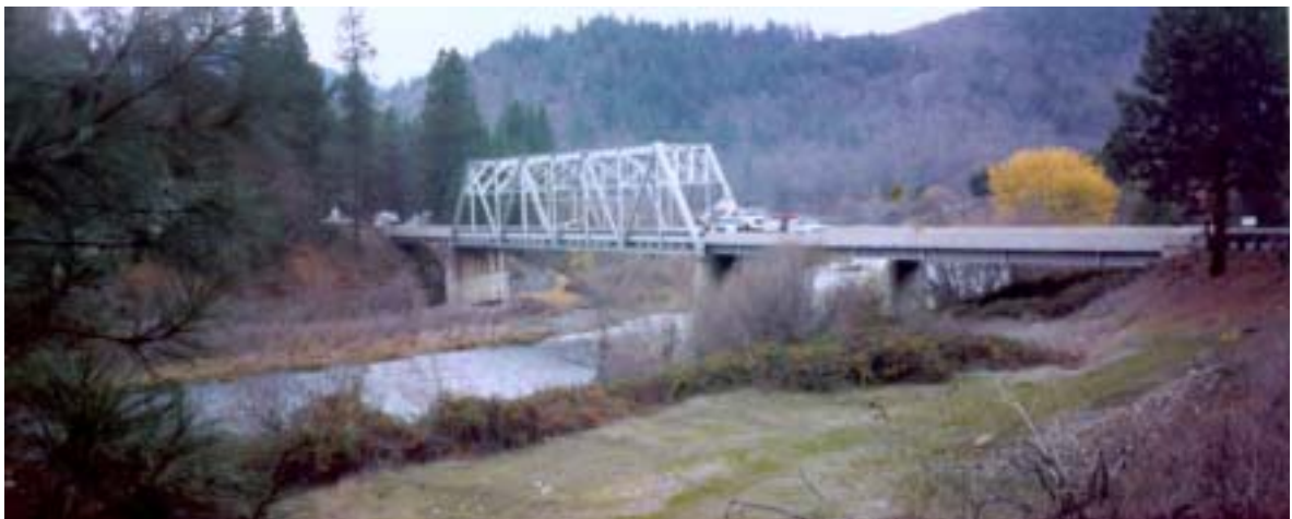
Figure 2-12: View of bridge 02-117 over the Klamath River, Horse Creek, CA.
