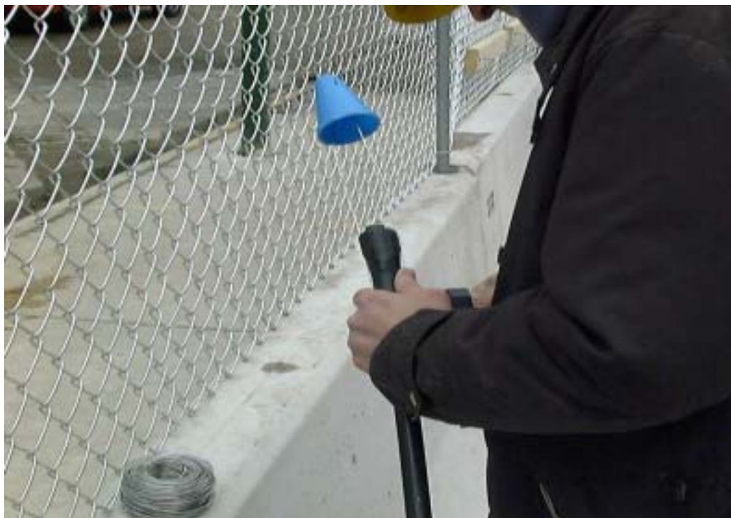
Figure 6-6: Installation of the penetration plastic cone at the end tip of a flexible braided cable at the Lurie Research Center, April 2002.
