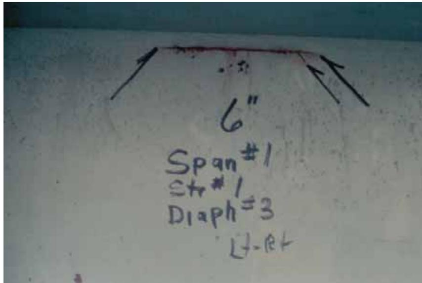
**Figure 4.2:** Fatigue crack marked as per the BIRM, after United States Department of Transportation: Federal Highway Administration (2006)
