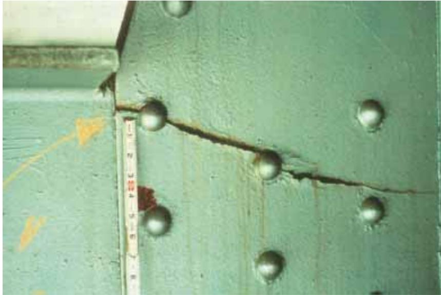
**Figure 4.1:** Fatigue crack at coped top flange of riveted connection, after United States Department of Transportation: Federal Highway Administration (2006)
