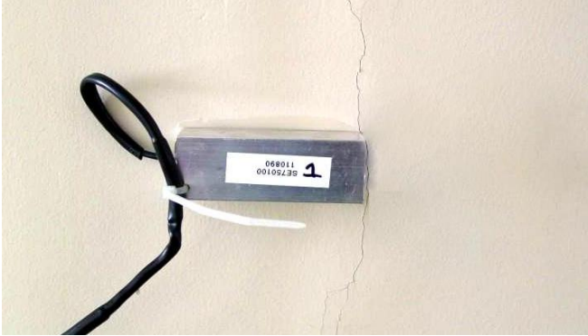
Figure 8: LVDT Body - Epoxied to Wall
