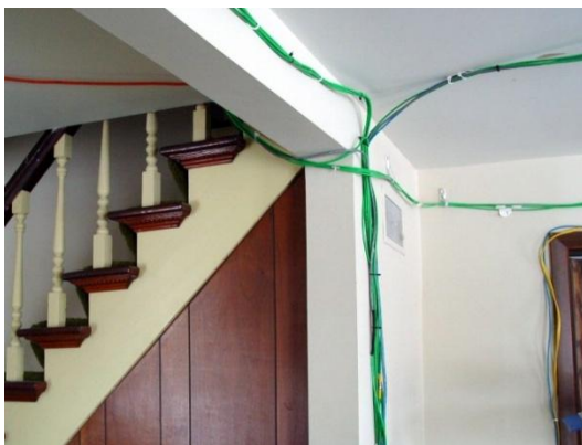
Figure 26: Example Wiring Between Floors
