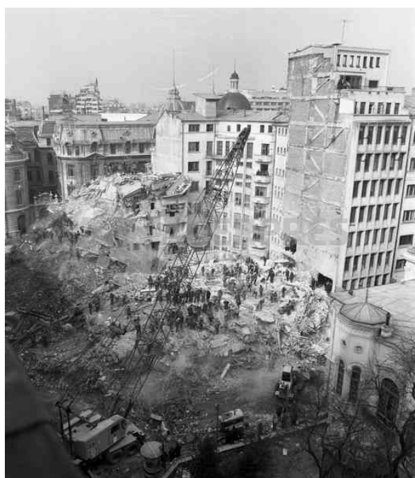
Figure 5. First-responders working at the completely collapsed Continental building, March 7, 1977. Workers found a six and a half year old girl 72 hours after the earthquake and a 19 year-old man in the basement 251 hours, or ten and a half days, later. The regime reported that of the registered residents 48% (76) had died, 23% (36) were missing, and 29% (45) survived. 43
