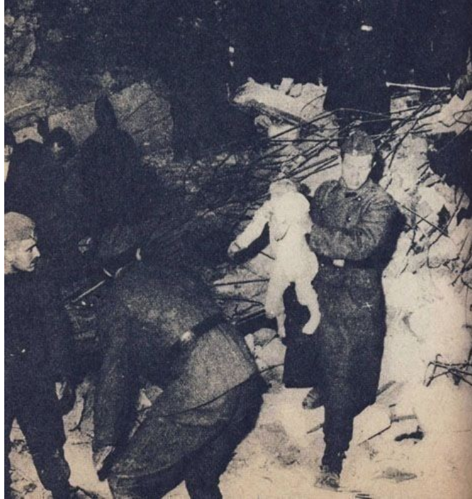
Figure 4. Regime officer removing a child from the rubble of an unidentified collapsed building in Bucharest. 26
