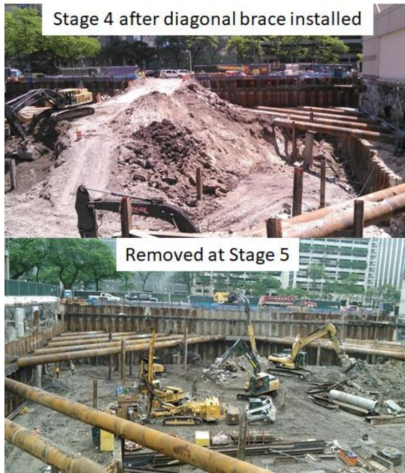
Figure 3.5 Access ramp along south wall
