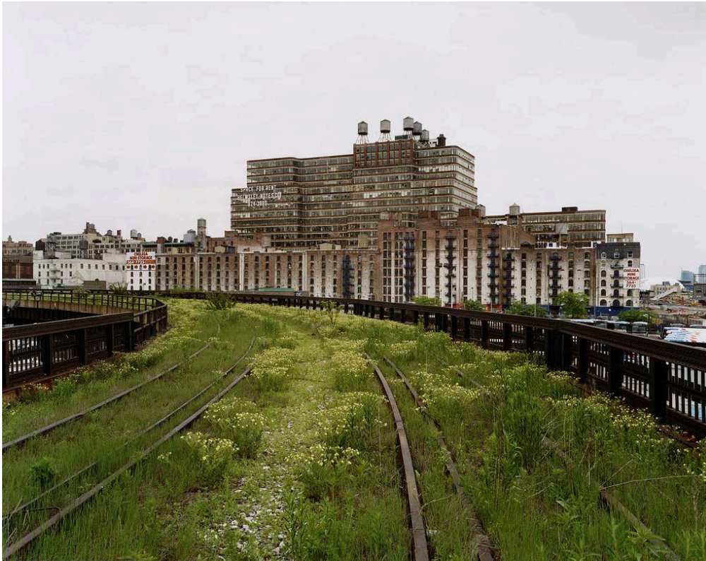
Figure 4.2: The High Line's original imbrication (photo by Joel Sternfeld, 2000)
