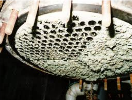
Figure 2: Fouled heat exchanger (regonline.com)
