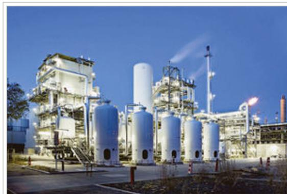
A hydrogen production plant with a box steam reformer
