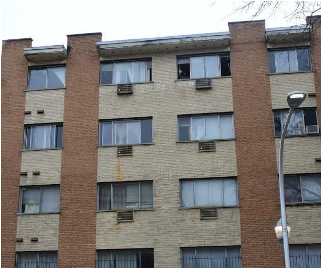
Figure 10. An image of mismatched and broken blinds in an apartment building
