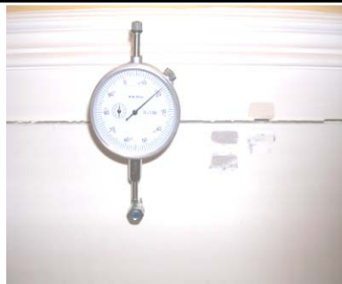
interior molding joint crack 2
